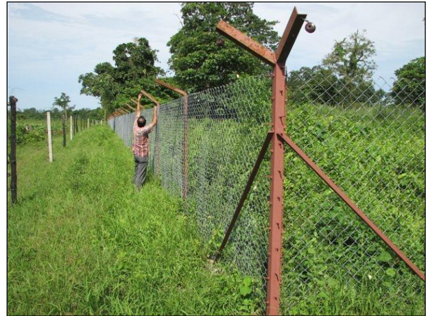
Perimeter security fence at Potasali
